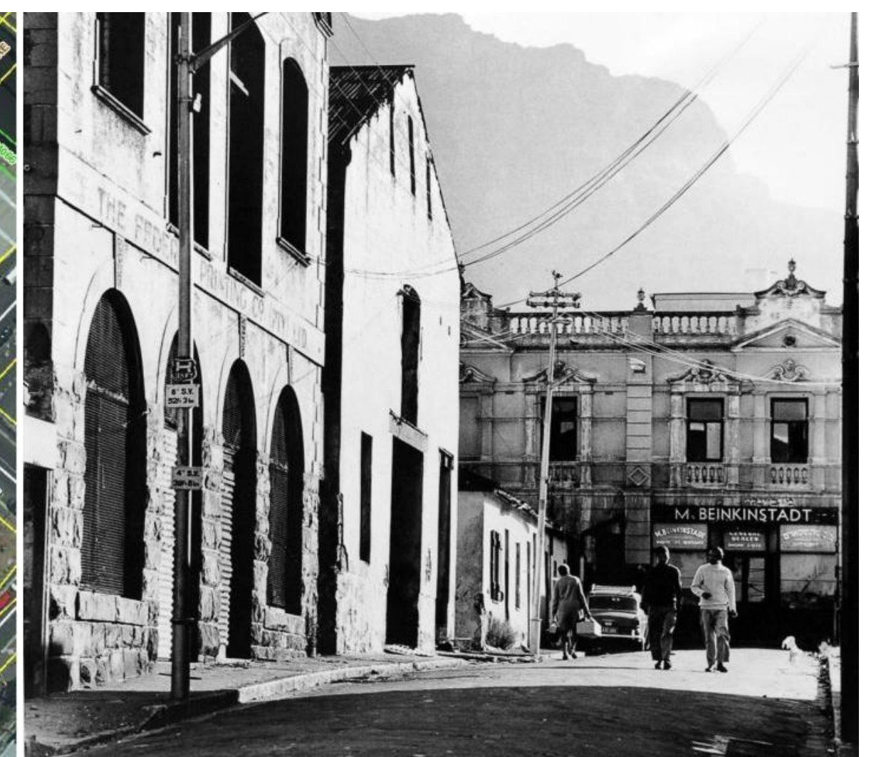
Cape Town/ District Six image in Glynndale St (previously Lamb's Lane) looking south towards Table Mountain with Beinkinstadt booksellers at the head of the road (Wissema, c.1970s).
