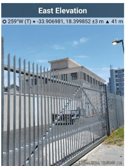
Photograph 7: Electrical substation on the site
