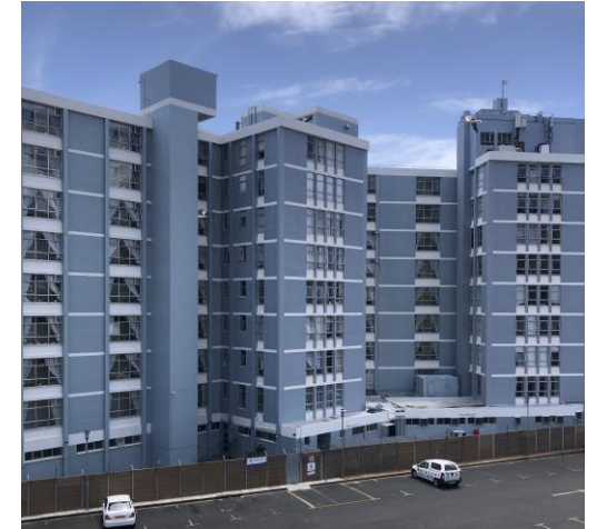
⑤ CPOA Building
