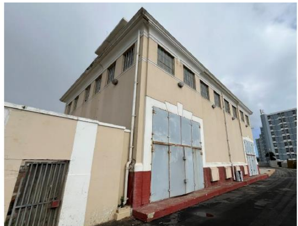
Electrical substation building.
