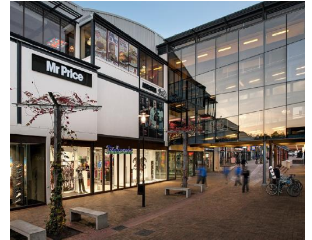
Eikestad Mall, Stellenbosch (Retail, Offices and Residential)
