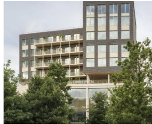
Multimodal Hub and Offices / DREAM + AIA Life Designers, Nantes, France
