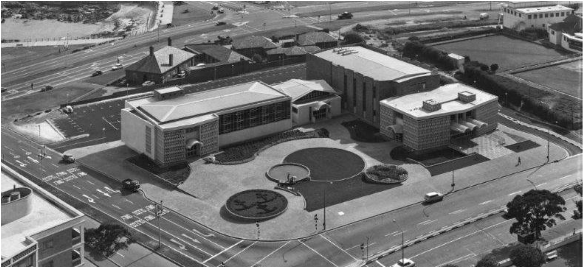
Figure 3.12: Photograph of the library and civic centre shortly after its completion (Source: CoCT) - the entire site is now fenced.
