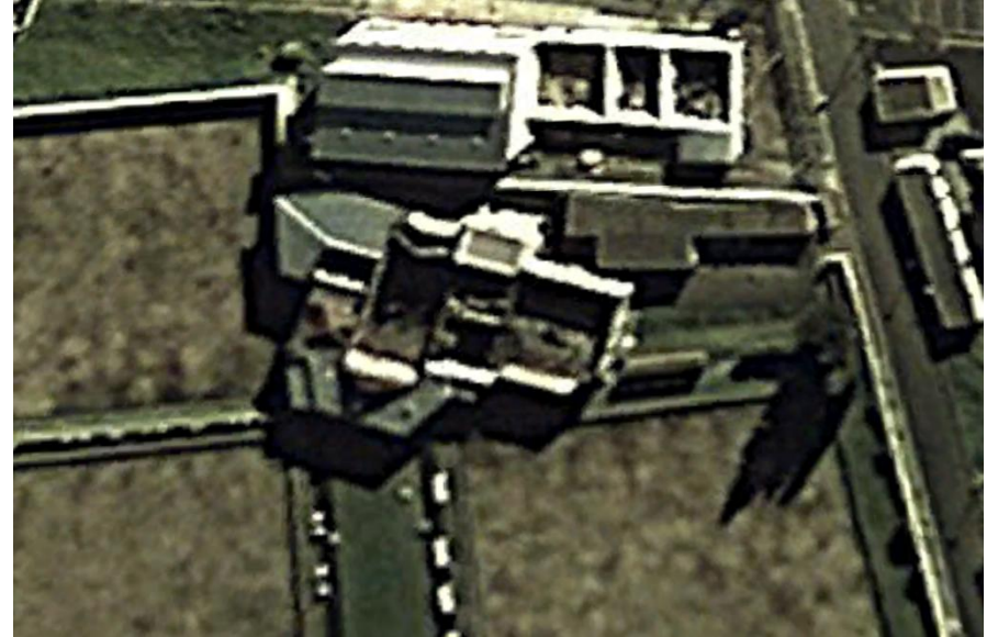
Figure 3.32: Google Earth image of the building after the fire of 2012 – dated 28 June 2013 (Source Google Earth Pro).
