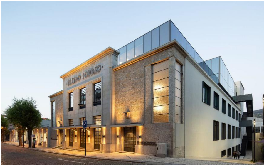
Figure 5.12: Rehabilitation of the Jordão Theatre, Guimarães, Portugal - Pitagoras Group
