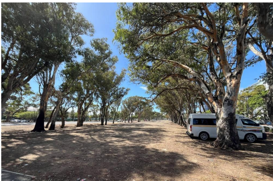
Figure 3.63: The eastern end of the site, looking east – fire damage is visible on the nearest tree trunk to the left (2025)
