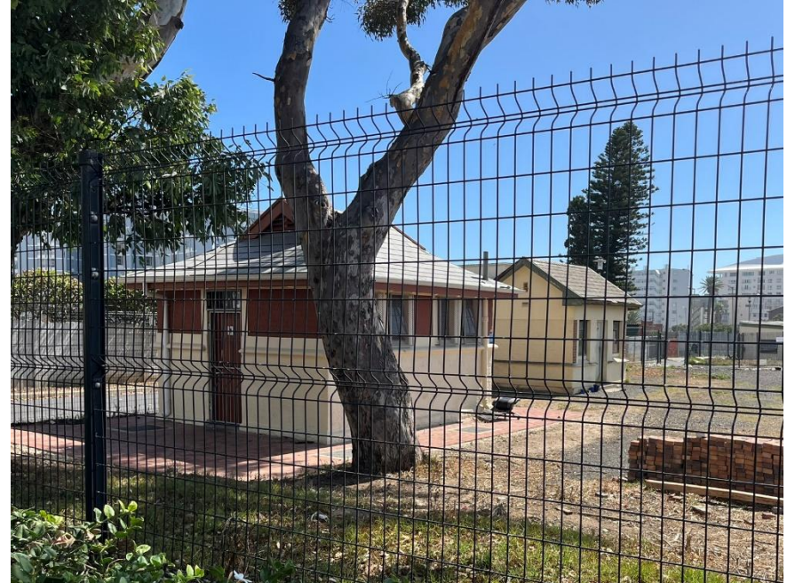
Figures 3.51 – 53: Outbuildings to second bowling club (Stadium)
