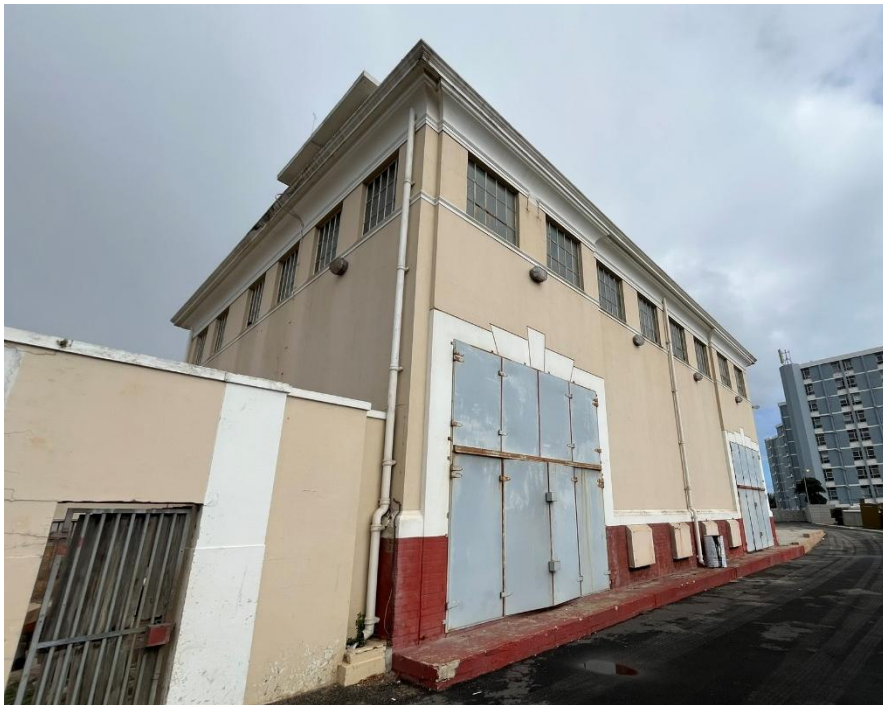
Figure 3.38: The substation building (2025)
