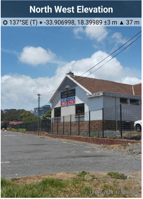
Photograph 12: Rear view of the Western Province Bridge Club
