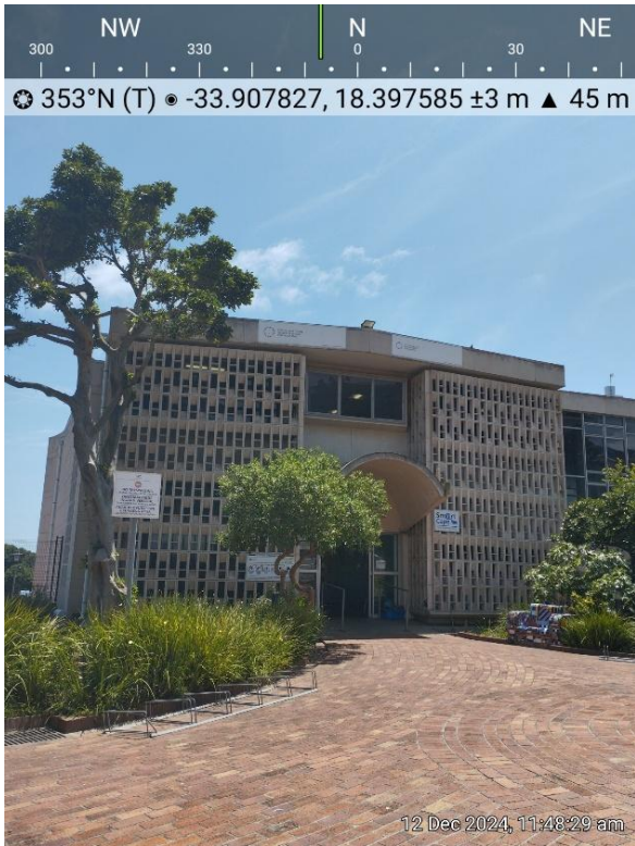
Photograph 1: Main entrance to the library through the forecourt
