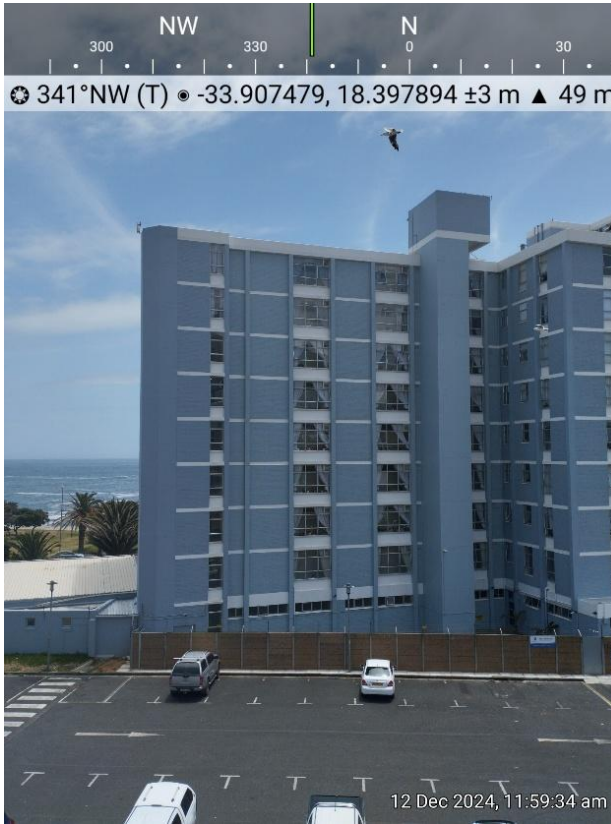
Photograph 7: Top view from the library roof of the Cape Peninsula Organisation for the Aged (CPOA), located northwest of the site (behind the library)
