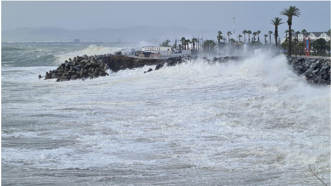
Figure 3-17: Overtopping of rock revetment at approximately 15:00 on 13 July 2020. Photo credit: Stephen Luger.
