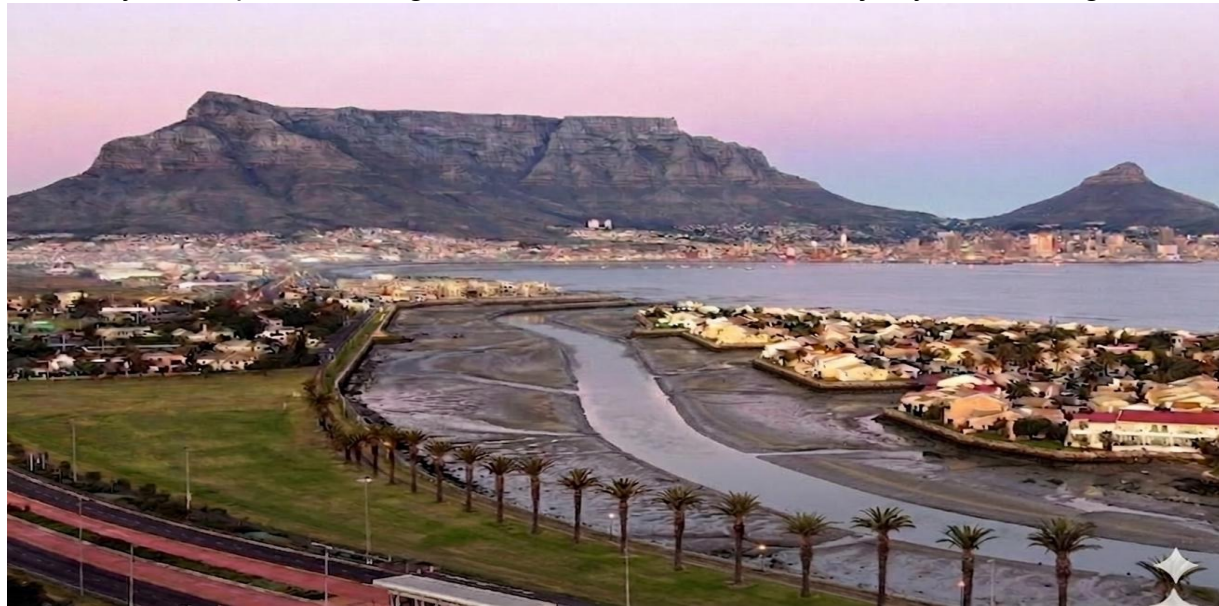
Expected majority view of the lagoon after the dredge – banks exposed for 16hrs a day.
